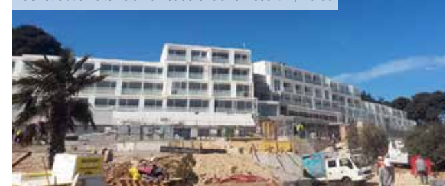
Construction site Valamar Isabella Island Resort 4*, Poreč
